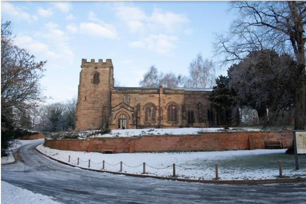
Photo 9: St Helen's Church (Grade 1)
